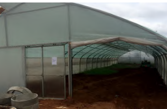
Single Span Tunnels
